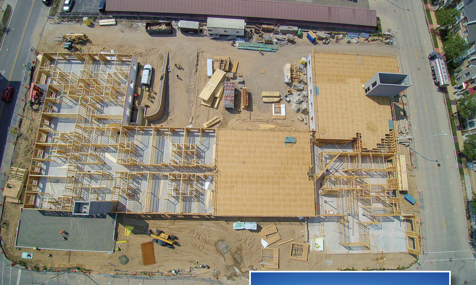
The Berkshire Muskegon, located in downtown Muskegon, Michigan, is a three-story senior apartment complex for residents 55 and older. Summit Building Services, LLC provided rough carpentry framing on the 92,000-square-foot building.
